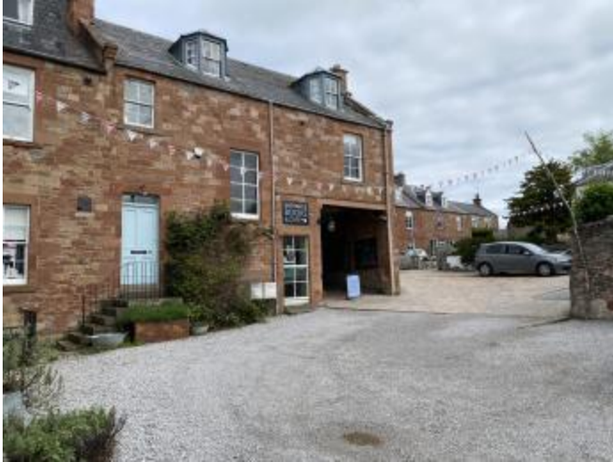
Exterior entrance, viewed from the car park, with archway to entrance. Gravel courtyard and route to carpark.
