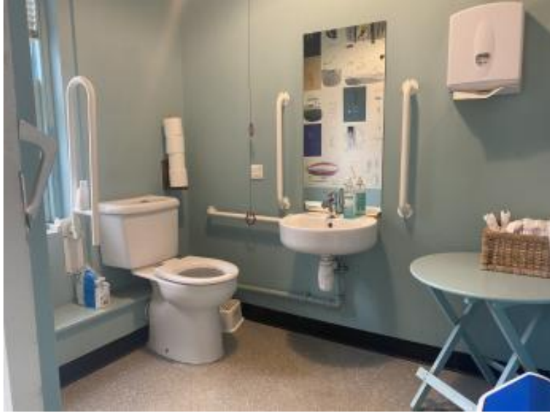
visitors toilet with handrails beside toilet and sink.
