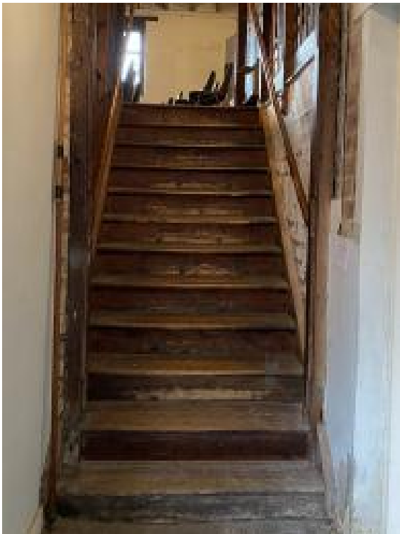
Stairs leading to the Barn space
