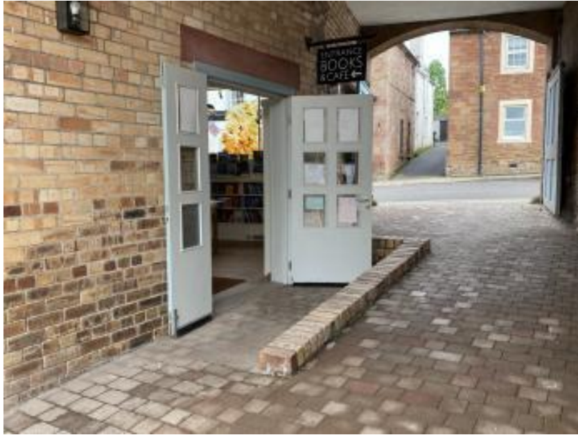
Accessible entrance with double doors open.
